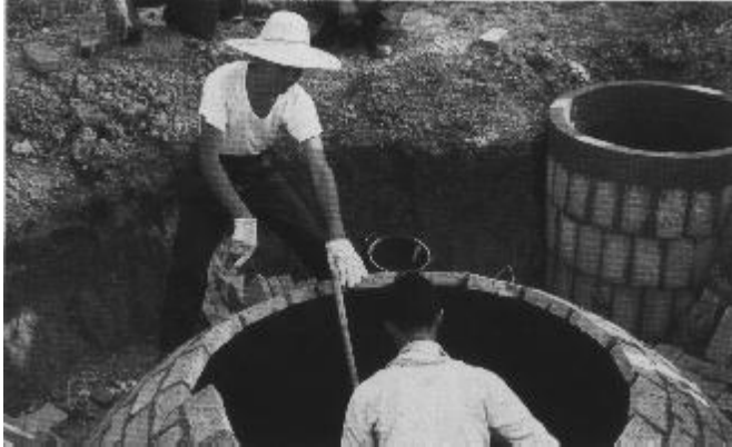
Figure 6: Installation of a Shanghai fixed-dome system near Shanghai, PR China Floating-drum plants
