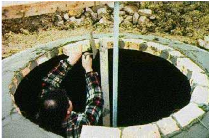
Figure 3: Fixed-dome plant in Tunisia. The final layers of the masonry structure are being fixed.
