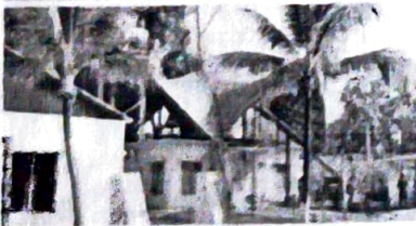
Bamboo Cafe Construction, Assam (Greenbam Infratech Pvt Ltd)
